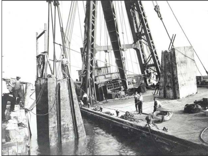
Figure 27. Setting of underwater concrete blocks for Contract 1, July 19, 1913.
