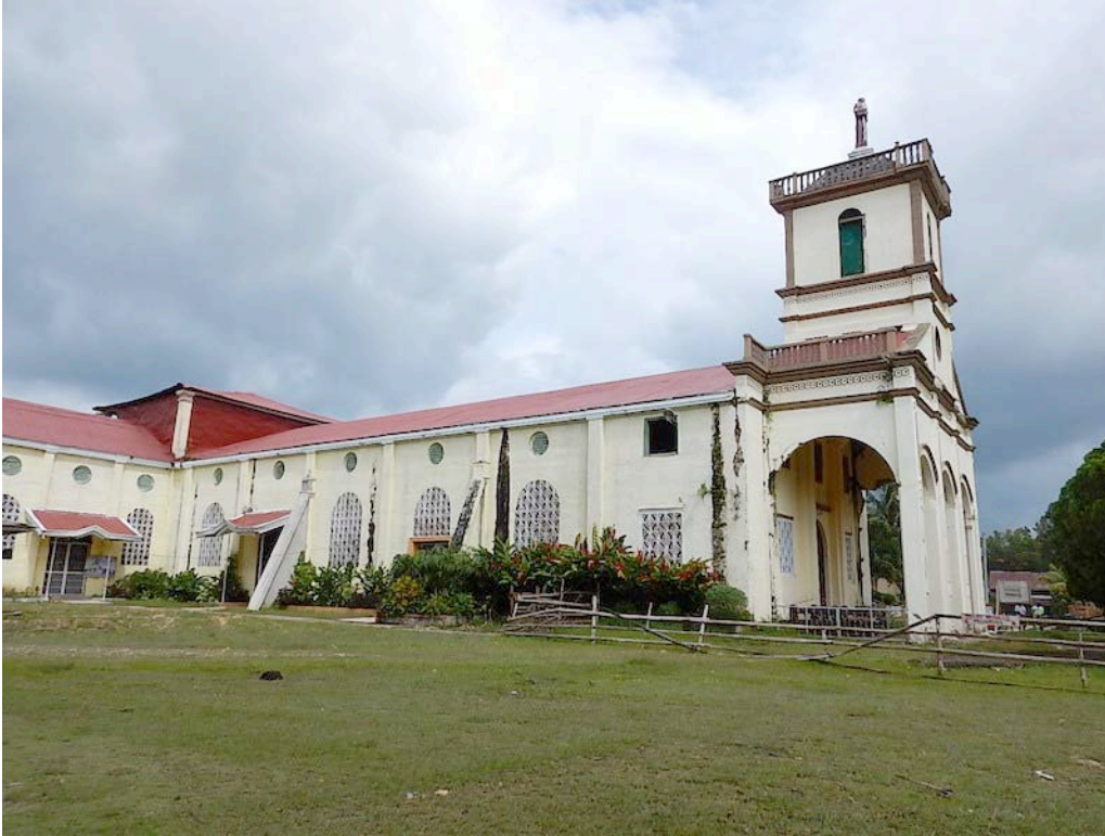
Figure 47. View of west elevation. Note the concrete buttresses that have been added to the original structure. The left buttress was recently constructed. See following figures for details.
