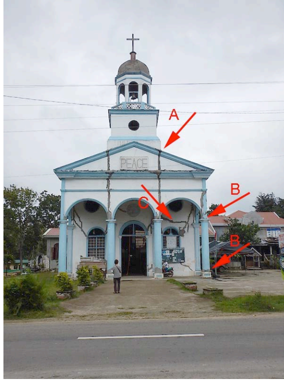
Figure 30. Front facade of the La Purisima Concepcion Church in Catigbian, built of reinforced concrete during the 1930s, and likely completed after WWII. The temple-front facade is typical of the churches in smaller towns of Bohol. Note recently patched vertical cracks at “A,” diagonal cracks at “B,” and cracks at the column top and base at “C.” See details and discussion in the following figures.
