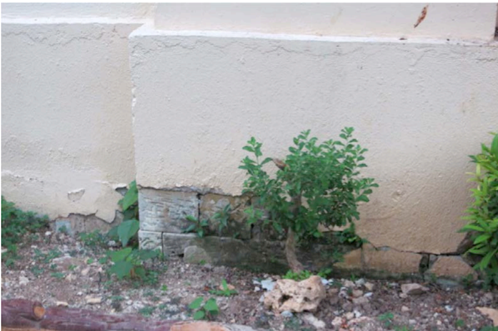
Figure 18. Exposed coralstone courses of the foundation wall, possibly dating from 1896.
