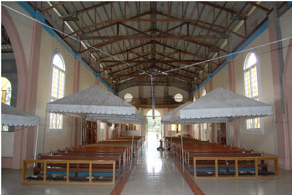
Figure 39. View of the sanctuary interior looking towards the entrance and choir loft above. Note the tents to protect from rainwater and bird guano.
