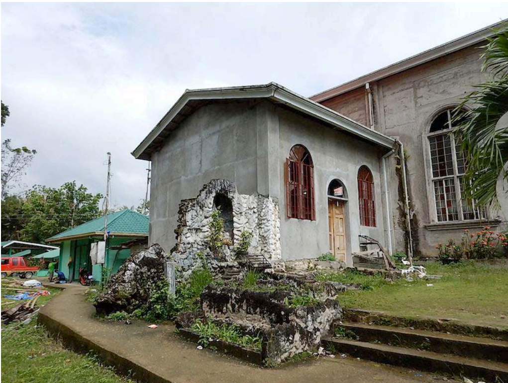
Figure 35. South transept, which was recently reconstructed.
