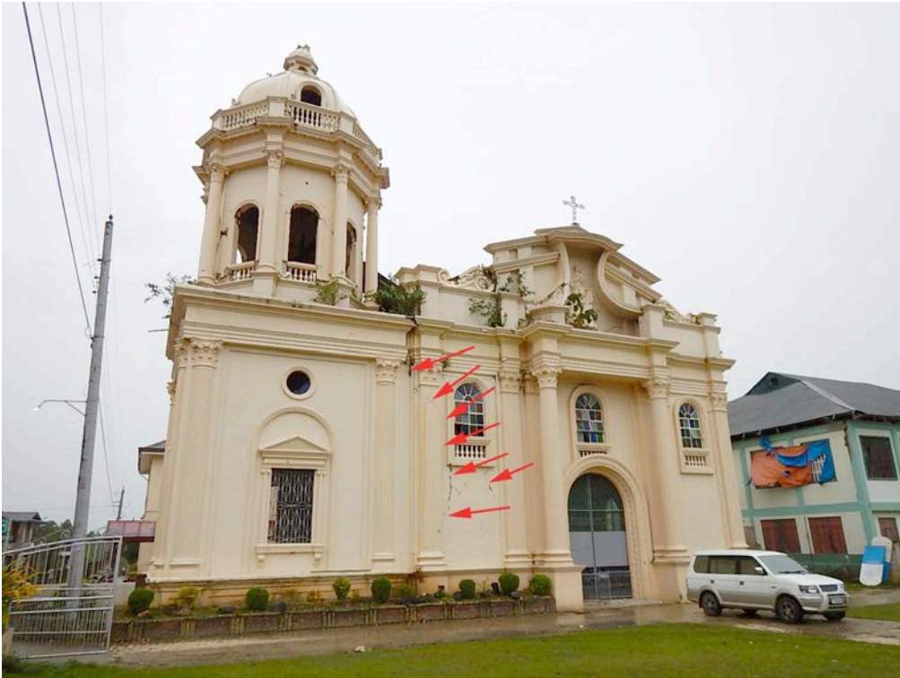
Figure 9. Front facade of Nuestra Señora del Rosario Church, Antequera, built of reinforced concrete over an older coralstone foundation. The front facade, which was constructed in the 1960s, is designed in the Baroque Revival style, with rococo features. There are cracks at the arrows, from rocking, and possibly pounding, from the bell tower. Note also plant growth at many locations above the cornice.
