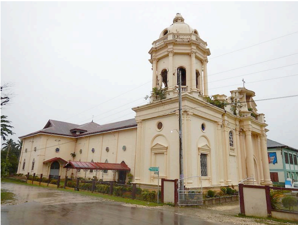
Figure 10. View of the northwest corner of the exterior, showing the bell tower cupola with its balustraded dome, and the north elevation and north transept.
