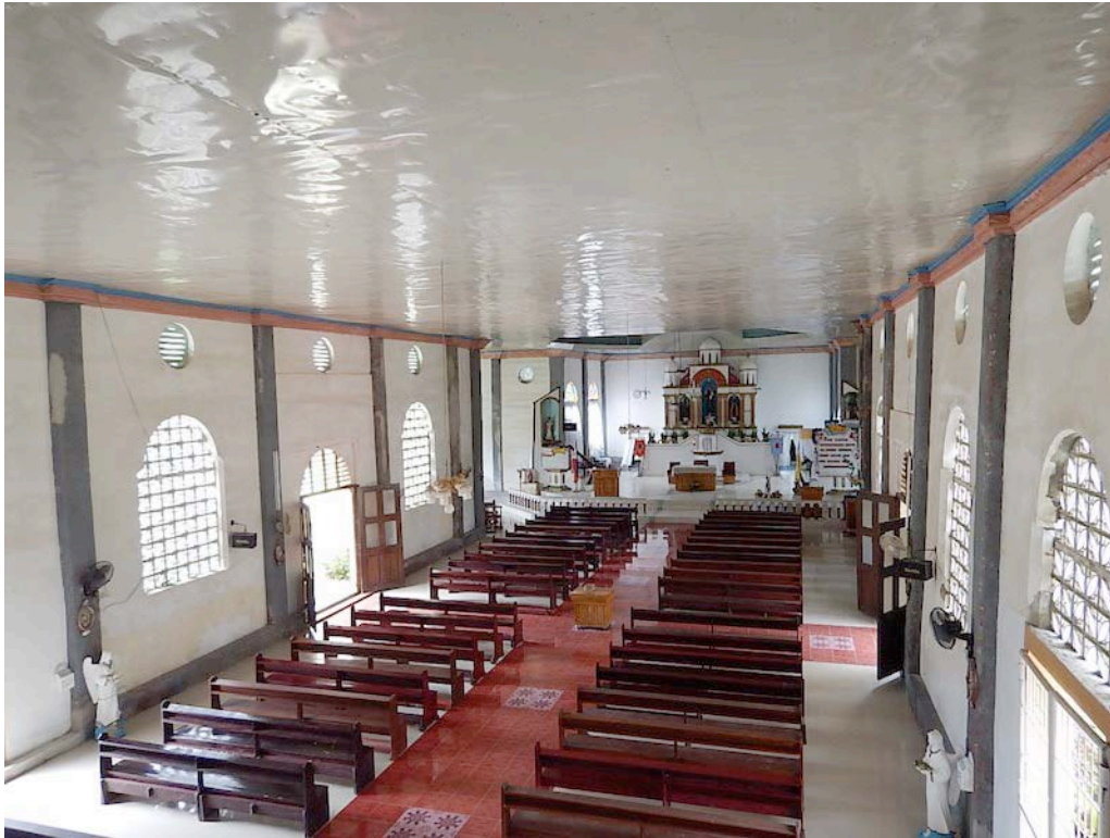
Figure 57. View of the interior from the choir loft. The ceiling appears to have been recently replaced.
